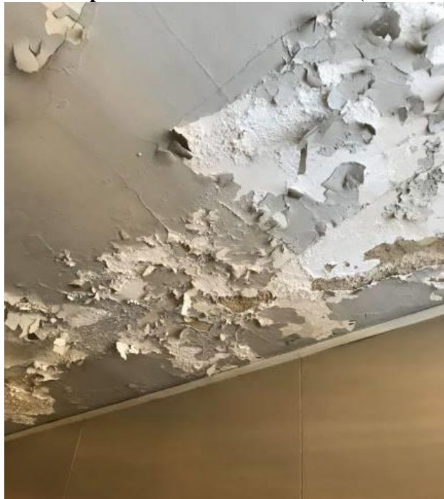
Mechanical Dept. – General Foreman Office (water intrusion)
