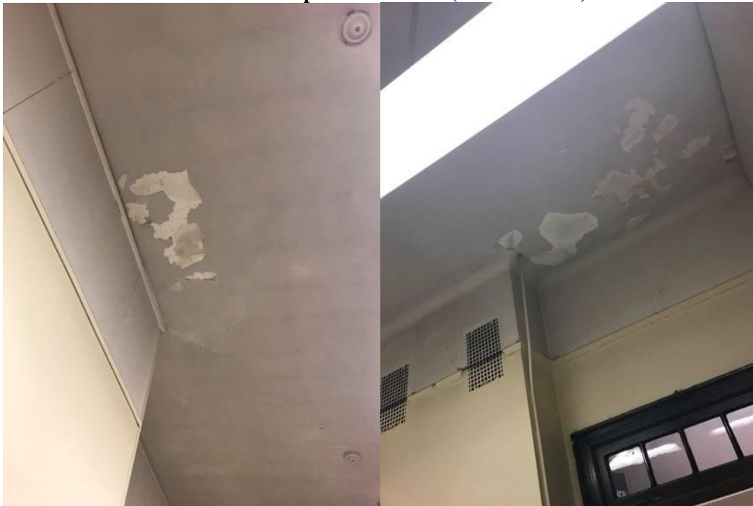
Mechanical Dept. – Clerk Area (water intrusion)
