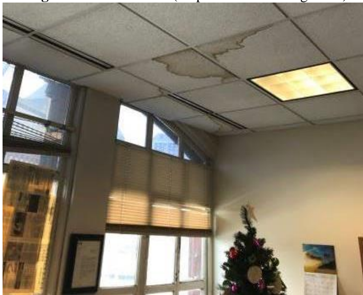
Engineer Lunch Room (suspected microbial growth)
