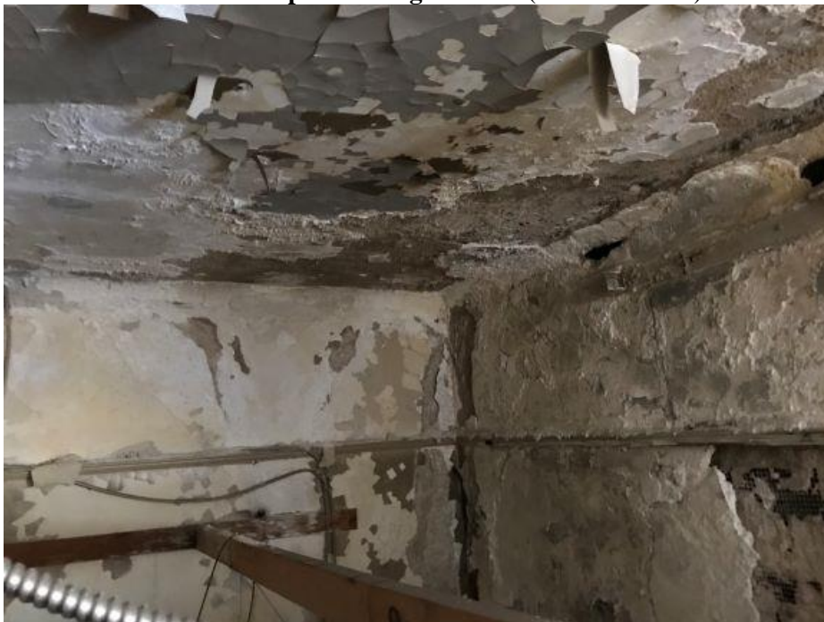
Mechanical Dept. – Manager Office (water intrusion)
