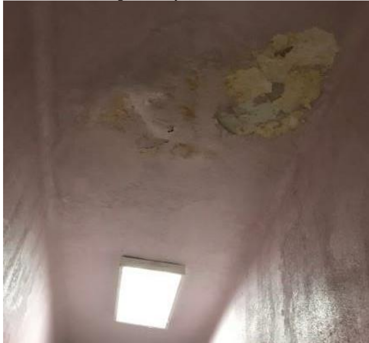
Mechanical Dept. – Clerk Area (water intrusion)
