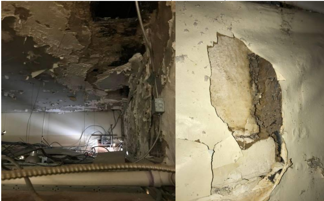
TCU Break Room (water intrusion)
