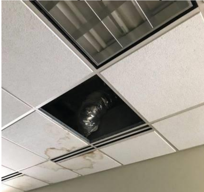
Engineer Lunch Room (suspected microbial growth)
