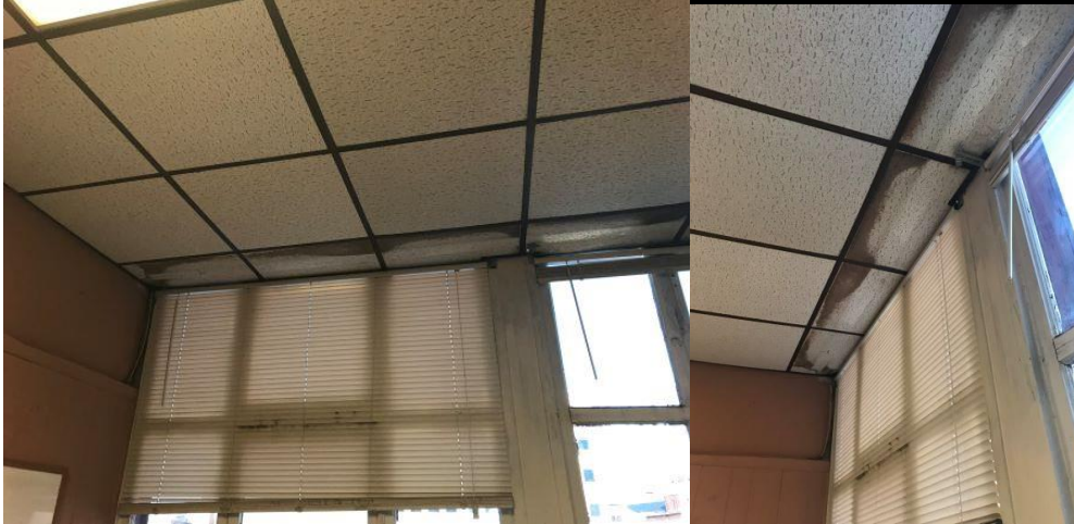
Mechanical Dept. – General Foreman Office (water intrusion)
