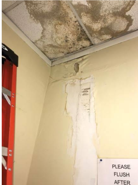
TCU Break Room (water intrusion)
