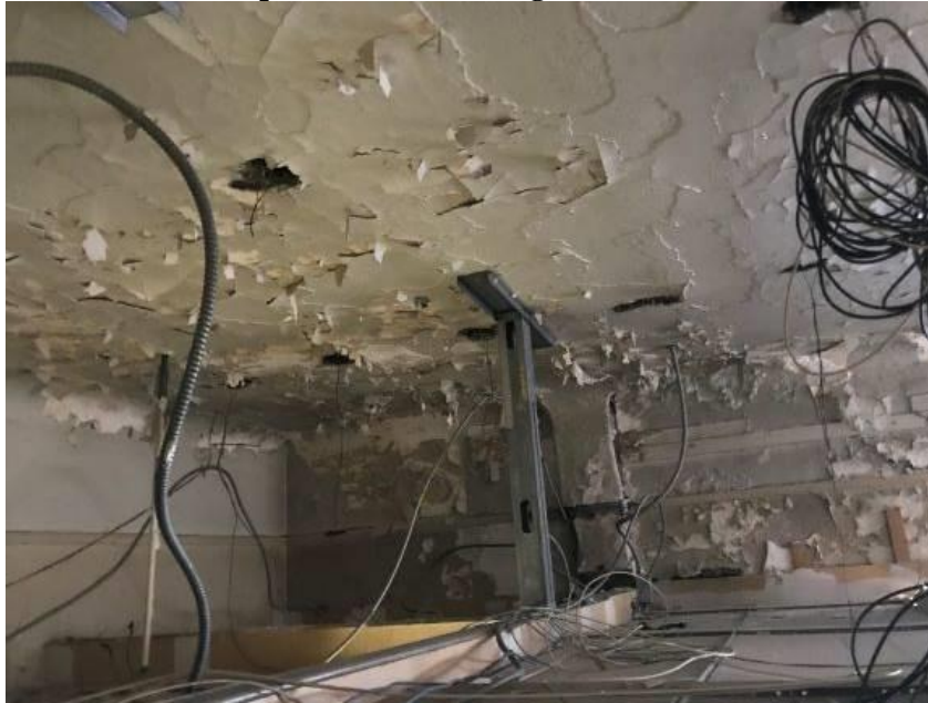
Mechanical Dept. – Manager Office (water intrusion)
