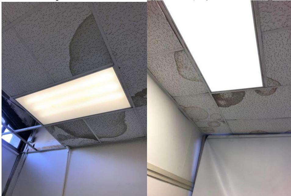
Mechanical Dept. – General Asst. Manager Office (suspected microbial growth)
